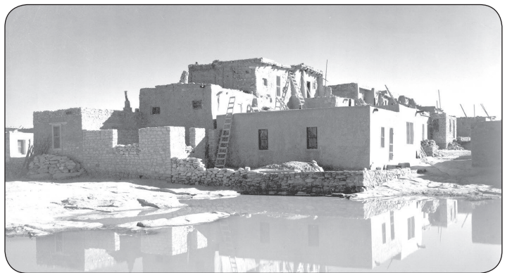
Native Americans in the Southwest used passive solar designs when building their homes.
